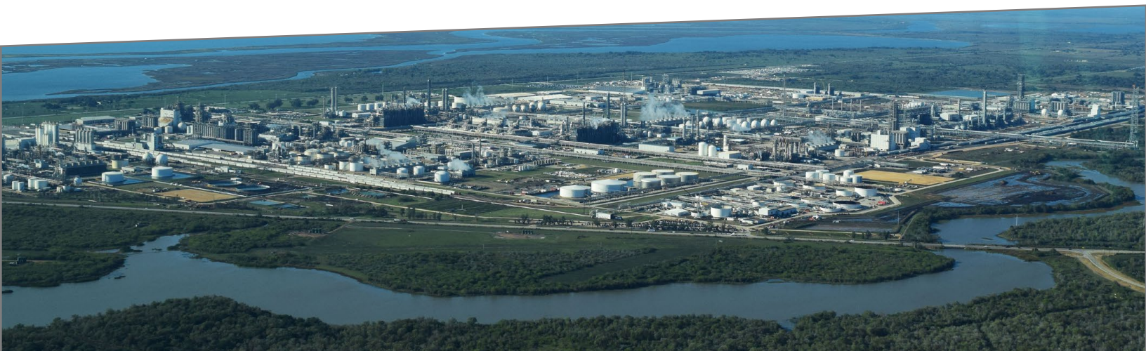
A PVC plastic facility in Point Comfort, Texas. Photo by Ted Auch, FracTracker Alliance, 2019. Aerial support provided by LightHawk
