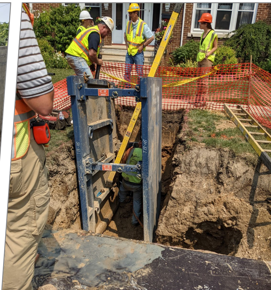
The bulk of the expense of replacing lead service lines comes from the costs of heavy machinery and labor, rather than from the cost of the replacement piping, regardless of what piping material is used. Lead service line replacement in progress in Stoughton, Wisconsin. Images by Casey Sweeney, courtesy of the Wisconsin Department of Natural Resources.
