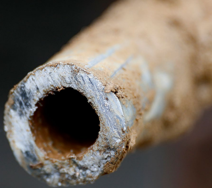
Lead pipe is shown after being replaced by a copper water supply line to a home in Flint, Michigan. (AP Photo/Paul Sancya)
