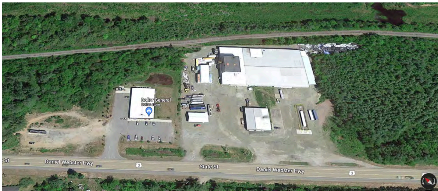
Prima America chemical recycling facility in Northumberland, New Hampshire. Source: Google Maps
