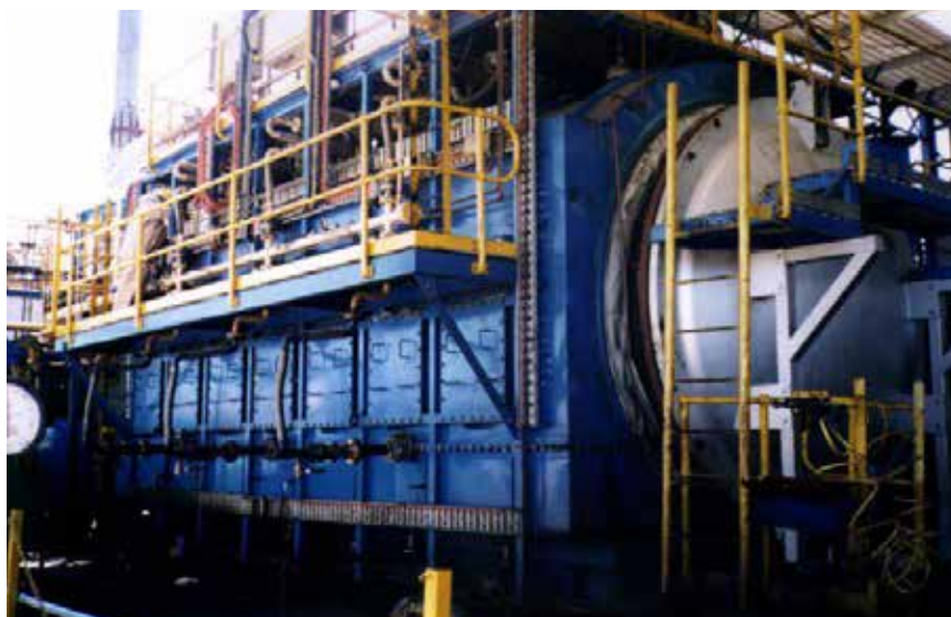
Figure 33. Thermal Reduction Batch Processor (TRPB) of the GPCR unit. Source: Hallett Environmental & Technology Group Inc. 2018
